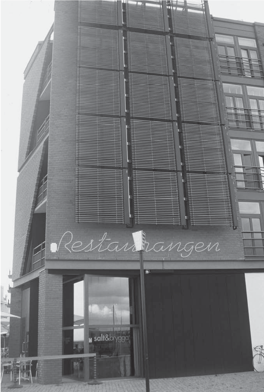
Figure 1 Vertical solar hot water panels in the sustainable planned district Vastra Hamnen, in Malmö, Sweden. (Photo by Tim Beatley.)
